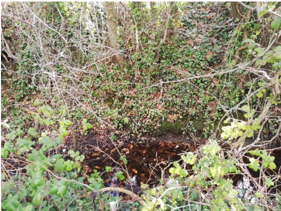
Plate 6-4: FW4- Drainage ditch
